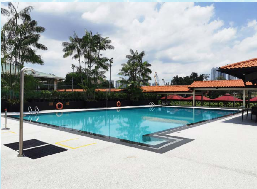
After: Our transformed swimming pool now complete with pebble-wash and timbered flooring on the deck areas.
