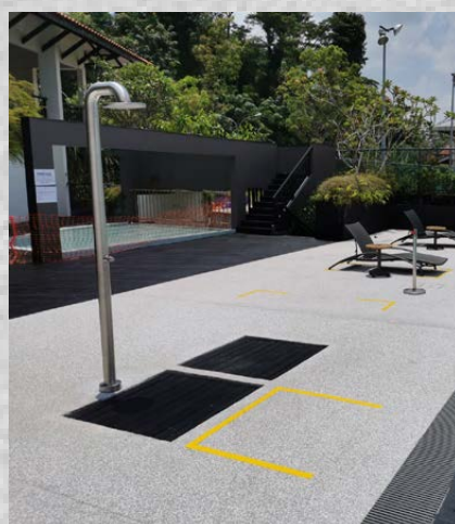
Swimming Pool: Rinse off areas: A clear demarcation line bearing in mind the 1 metre safe distancing
